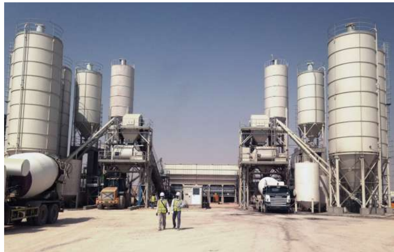
Ryadh, Saudi Arabia: Railway metro project
