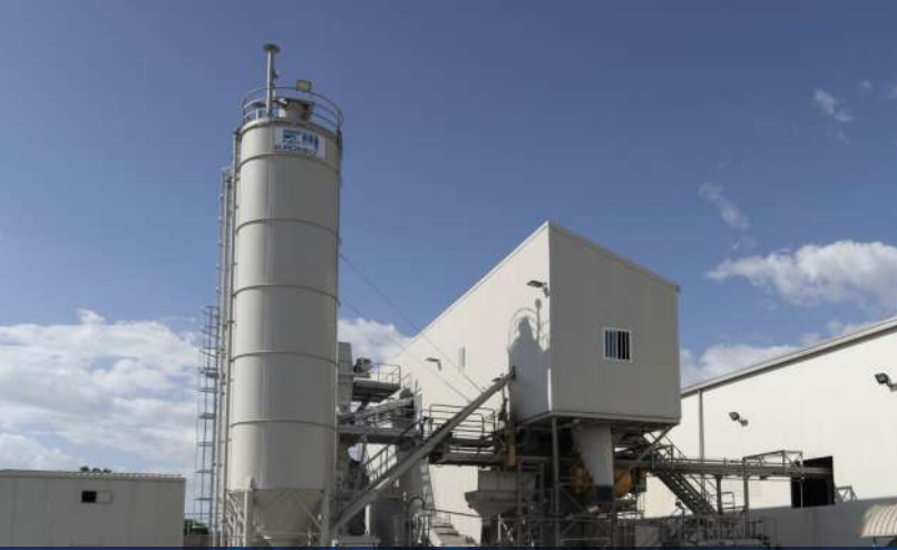
Catania, Italy: pre-cast factory for HS railway elements
