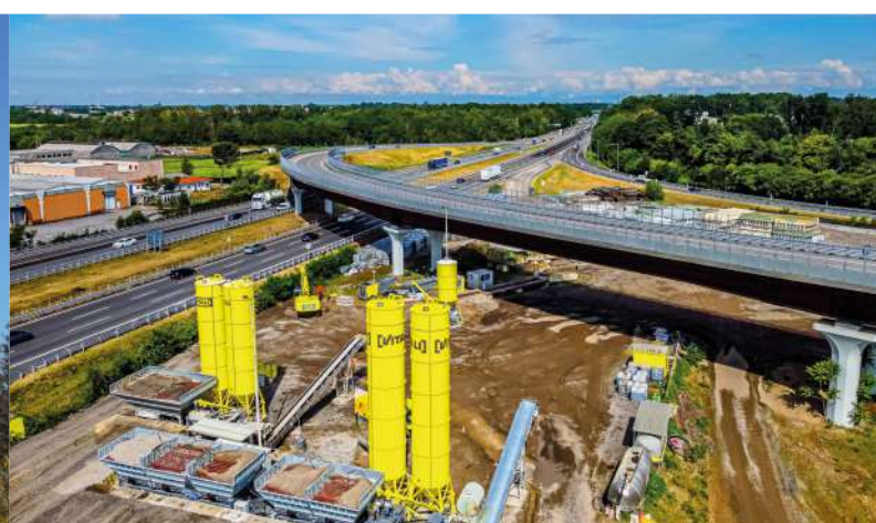
Milan, Italy: Readymix and Cement Mixture for Highways
