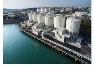
Pneumatic pipes facilitate the following of special routings and can be used either in dense or fluid phases.
