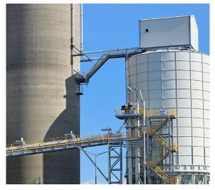
To compensate the height requirement, it is common to use a bucket elevator in combination with airslides.
