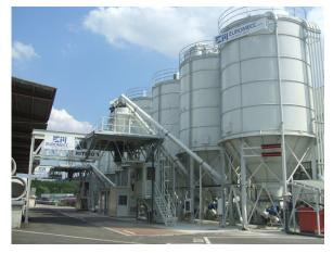
Screw conveyors guarantee high-flexibility from an operational point of view. They are popular in bulk loading stations, allowing silos to be installed at ground level without big frames or carrying structures.
