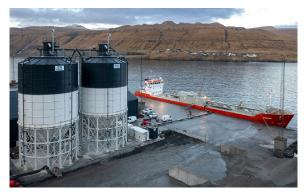
Pneumatic transport is the easiest means of transportation when cement is delivered by a self-discharging vessel. It minimises the infrastructure and protects the customer in the event of demurrage costs.
