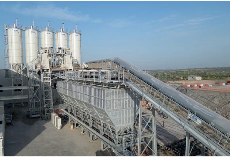
Assembly phase of concrete batching plant
