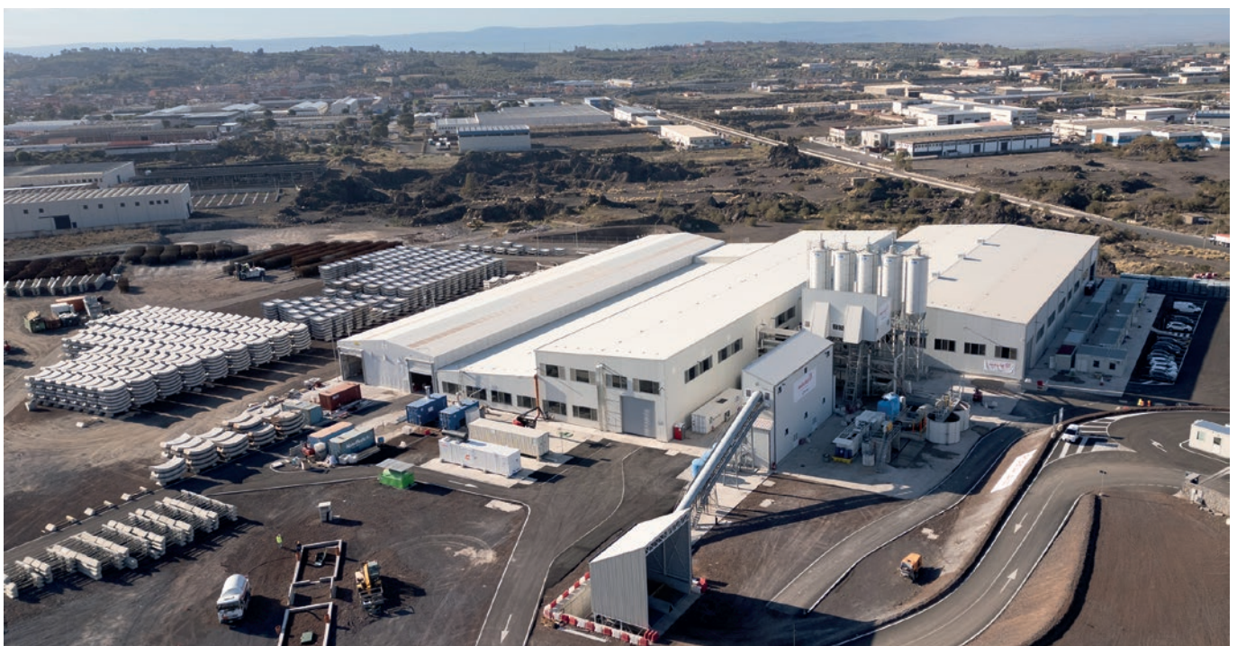
Production area of segments
